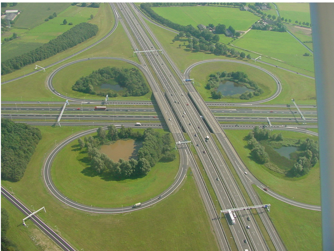
Figure 4.3: Aerial photo of the 'Beekbergen' cloverleaf junction – tilted angle.
